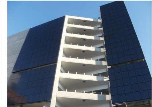
Figure 68: Example of mounted PV surfaces
