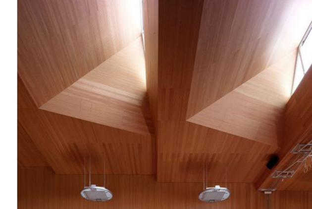
Figure 74: Example of skylights
